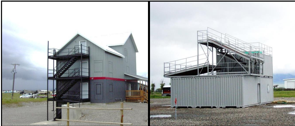
Figure 88: Sample Training Facilities
